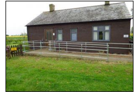
Darlow Farm Cottage NOW
